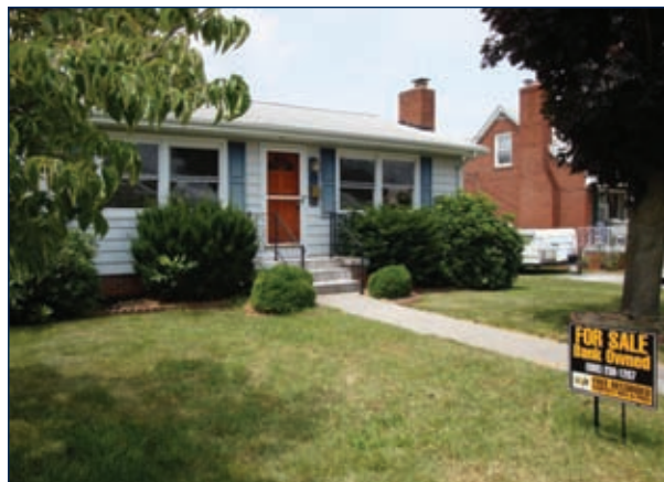
This foreclosed home in Front Royal, Va., was targeted for rehabilitation under the federal government's Neighborhood Stabilization Program, which helps communities struggling with foreclosure. The Richmond Fed visited the area in July 2009 as part of a case study conducted with the Cleveland Fed that analyzed how communities were implementing the program.
