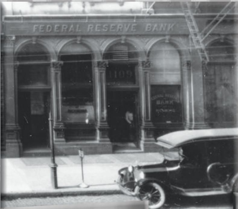
1914: The Richmond Fed's first building at 1109 E. Main St.
