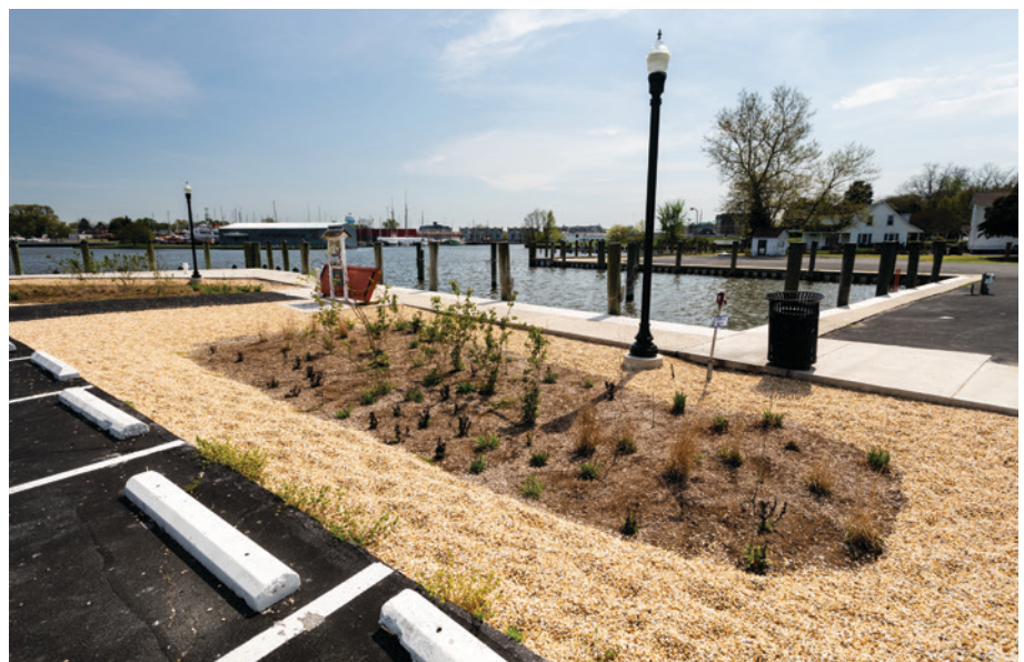
A rain garden at Long Wharf Park captures and filters stormwater pollution before it reaches the Choptank River in Dorchester County, Md.
