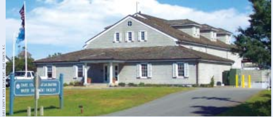
Parts of coastal North Carolina depend on desalted groundwater to supplement their water supply. Dare County, N.C., has built three desalination plants over the last 14 years to support their burgeoning residential development and tourist trade.
