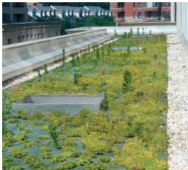
Completed in October 2003, this retrofit living roof atop the Arlington County Government Center is filling in quickly. The county also plans to top a community center and a fire station with sections of vegetative roofing.
