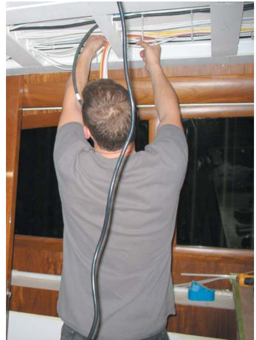
It takes a lot of wiring to provide the electronics that customers expect.
