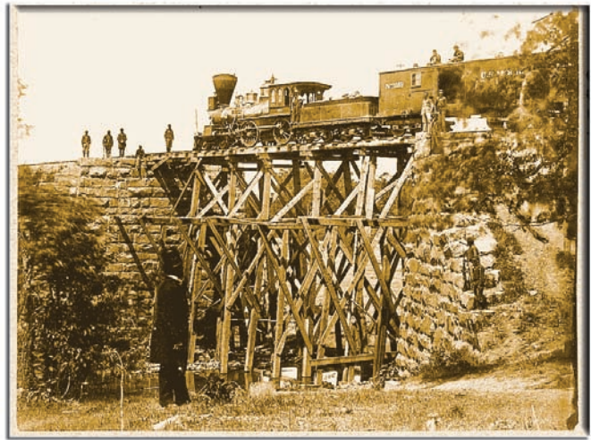
A bridge on the Orange & Alexandria, Va., Railroad, as repaired by Union army engineers ca. 1865.
