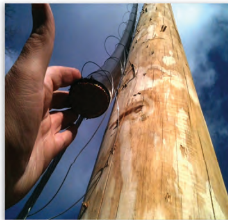
A Frontier Communications’ employee surveys the damage left behind by copper thieves in West Virginia. The company has replaced 38,000 feet of stolen cable since August 2011.
