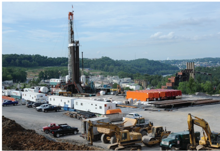
Northeast Natural Energy’s shale gas drilling operation is located in the Morgantown Industrial Park in Monongalia County, W.Va.
